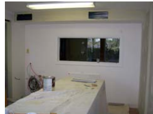
Empty Control Room
