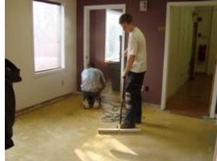
Sweeping before laying floor
