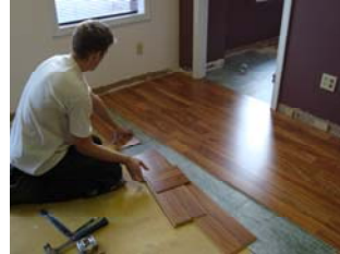
Laying down flooring
